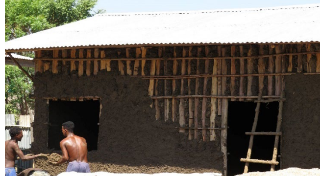
4. Classrooms under construction
